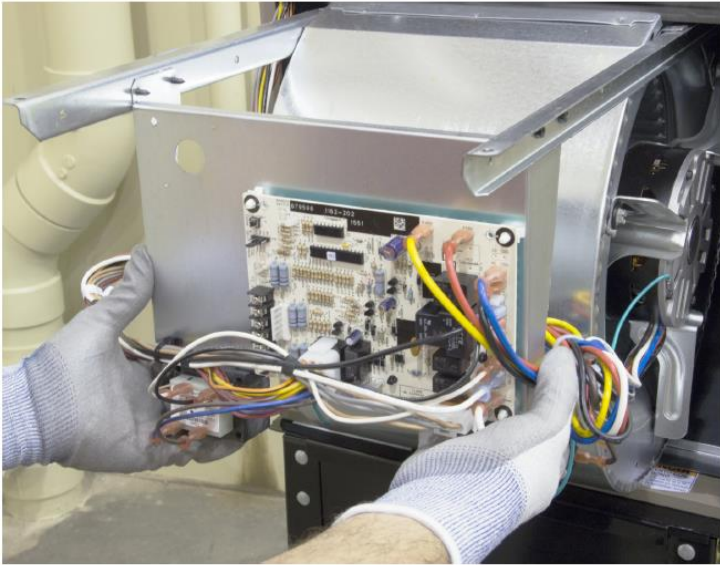
Slideout Blower Assembly
