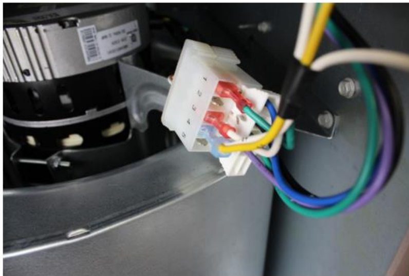
Standard ECM Low Voltage Connections
