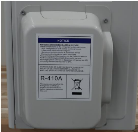
HMH7 Refrigerant Line Access Cover
