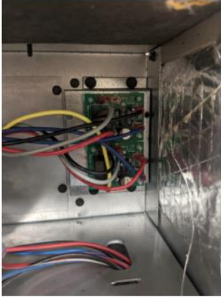
HMH7AK001 Blower Relay Kit Installed
