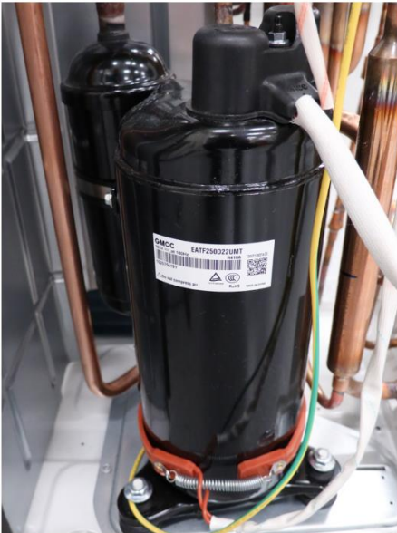
The HMH7 Twin Rotary Compressor with Accumulator and Crankcase Heater
