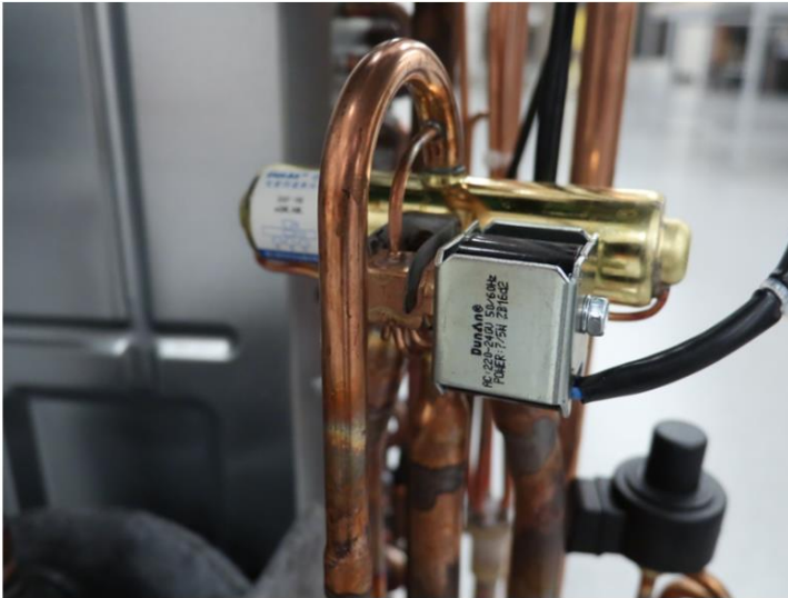
Reversing Valve (4-Way Valve) Note: The voltage applied to the reversing valve coil is line voltage (240 volt)
