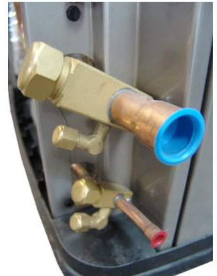
Liquid Line & Suction Line Service Valves
