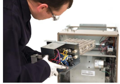
Electric Heat Kit Installation
