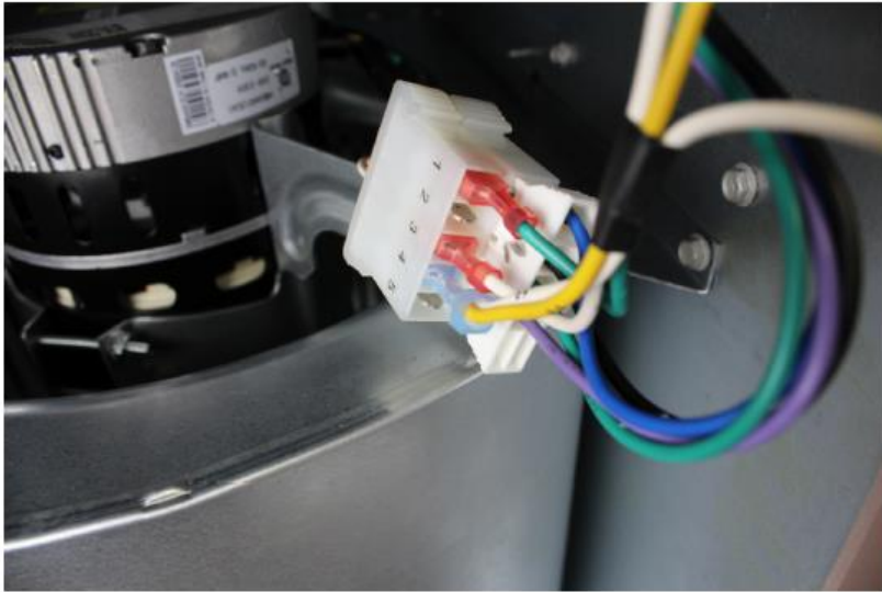
Speed Selection Plug: Standard ECM Motor
