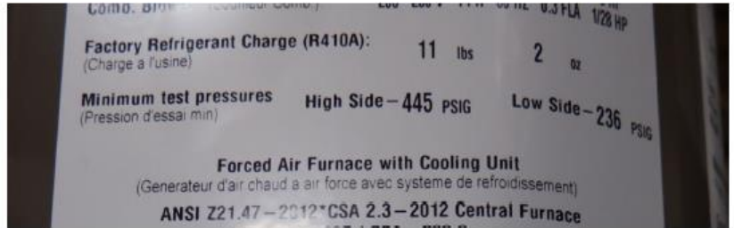
Rating Plate: Refrigerant Charge Data
