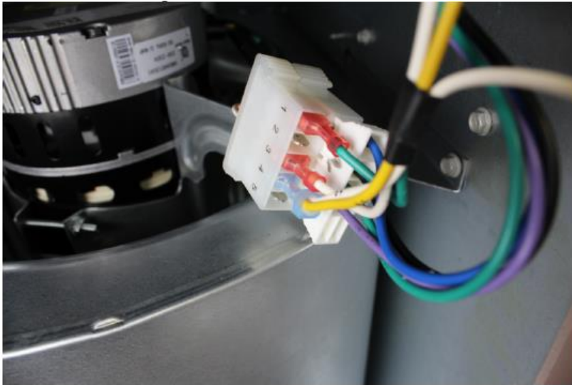
S-ECM Blower Motor Speed Tap Selection
