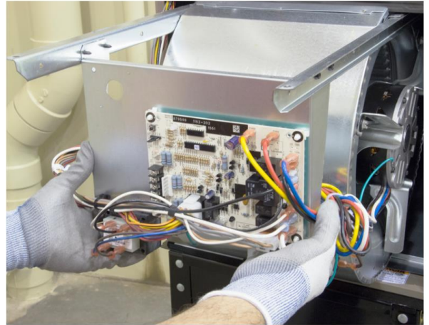
Blower Assembly Removal
