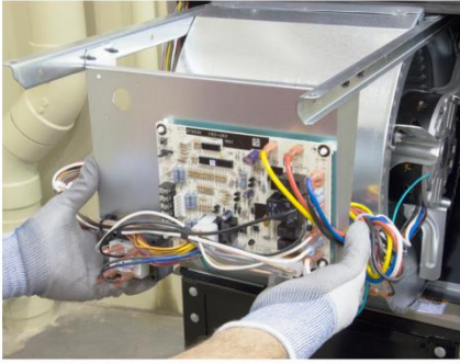
Blower Assembly Removal
